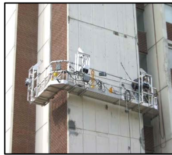
Powered Suspended Scaffold
